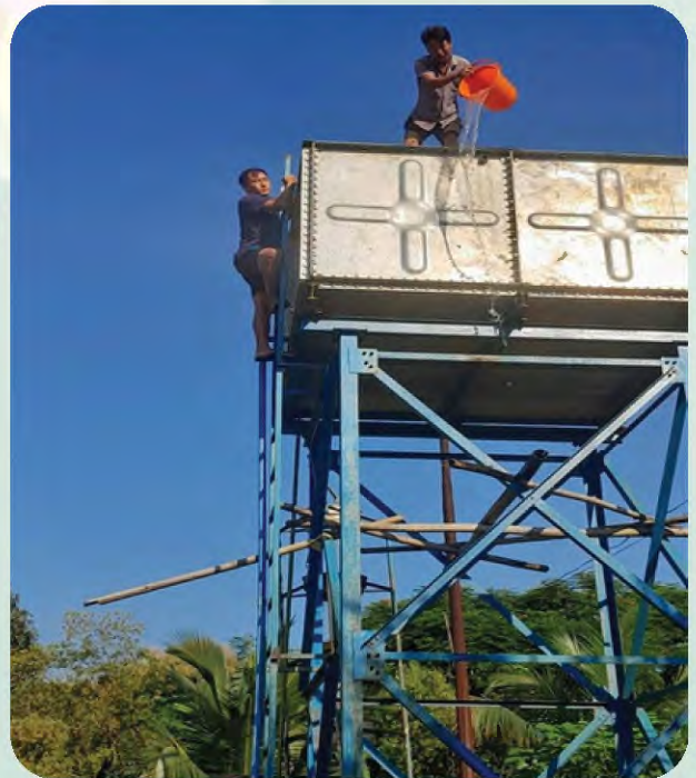
Cleaning of water tank in Dimapur, Nagaland
