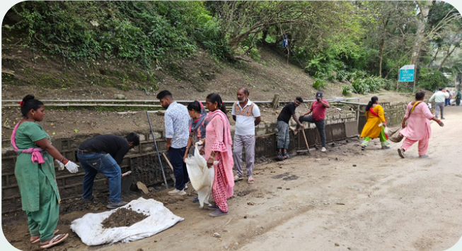
Cantonment Board Subathu and residents in Solan district, Himachal Pradesh, joined Swachhata Hi Sewa 2025, clearing clogged drains to improve cleanliness and safety
