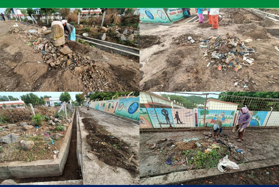
An underground sump was created to collect drainage water, due to the existing poor construction of Drainage (or) different levels of drainage systems, which were built, in two different periods.
